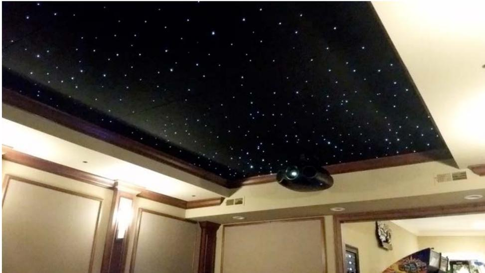
Here at EHTS we design and install every fiber by hand at your location. This ensures the most realistic looking night sky. We install fibers of four different diameters to simulate stars at different distances. Are digital light generator also emulated twinkling stars.
